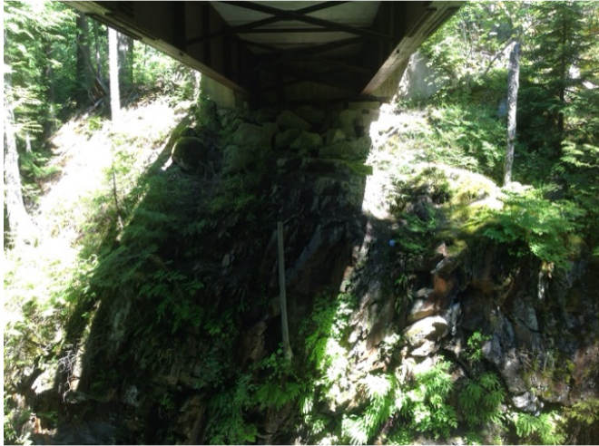
Right Bank Abutment when facing downstream
