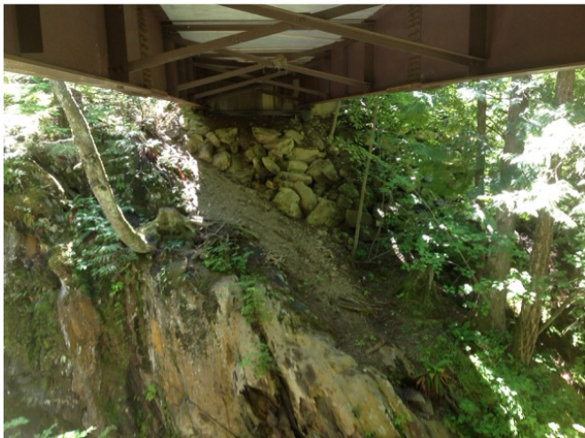
Left Bank Abutment when facing downstream
