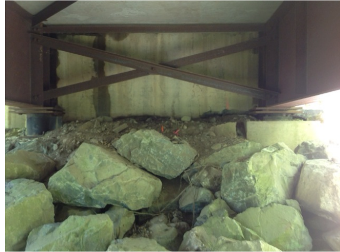
right bank bearing
